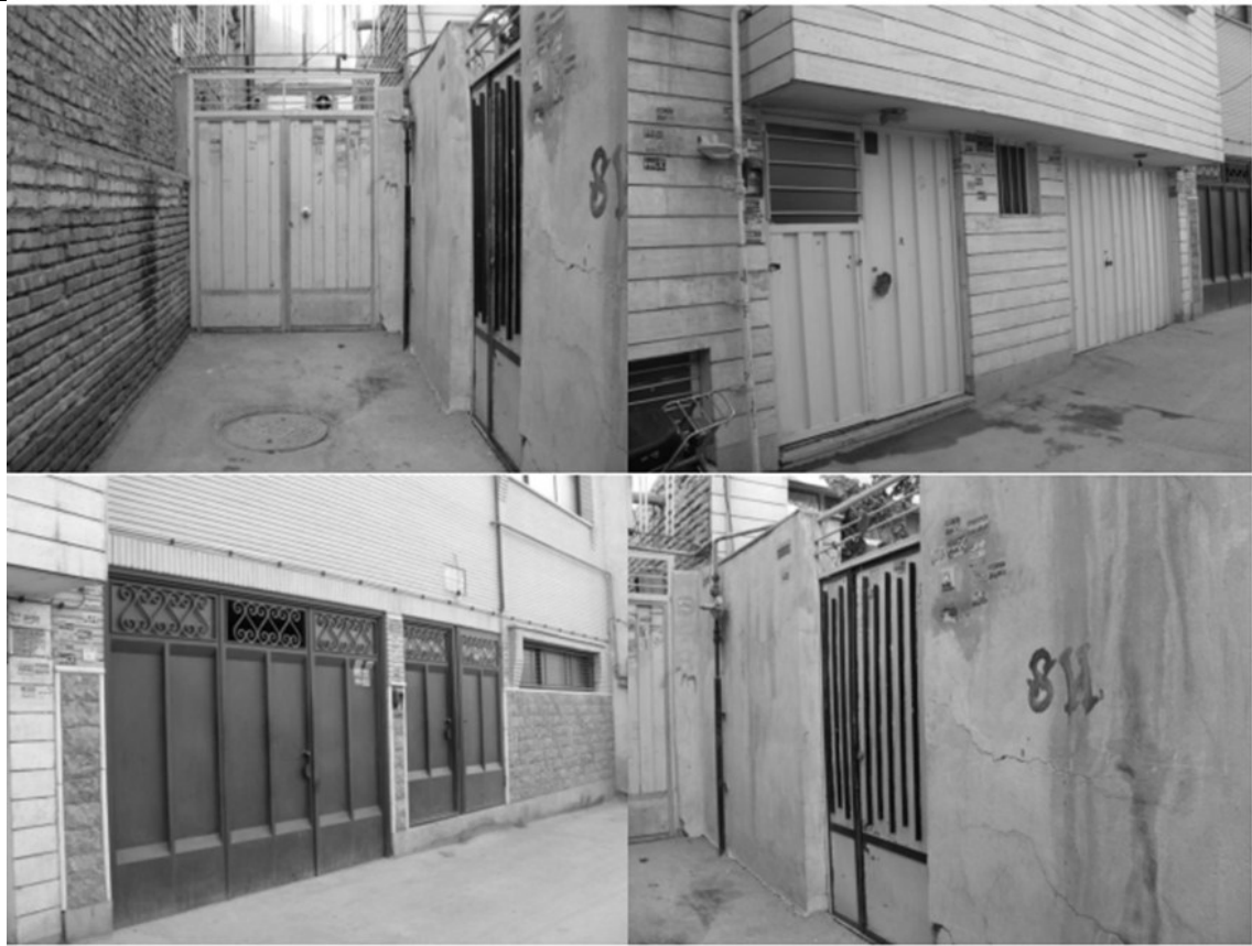
Problem 6: Sticking advertising Stickers on doors and façade walls. Solution: Design advertising boards.
