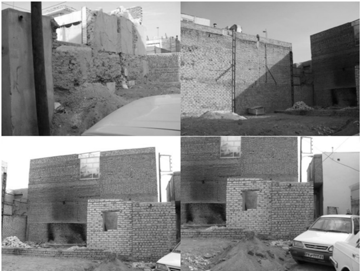
Problem 7: The dilapidated space is being turned into a parking lot and a garbage dump. Solution: Design a parking lot and empty the garbage.
