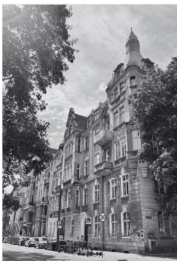
Fig. 4. View of the façades of tenement houses at 55–60 Matejki Street, 2025 (photo by the author).
