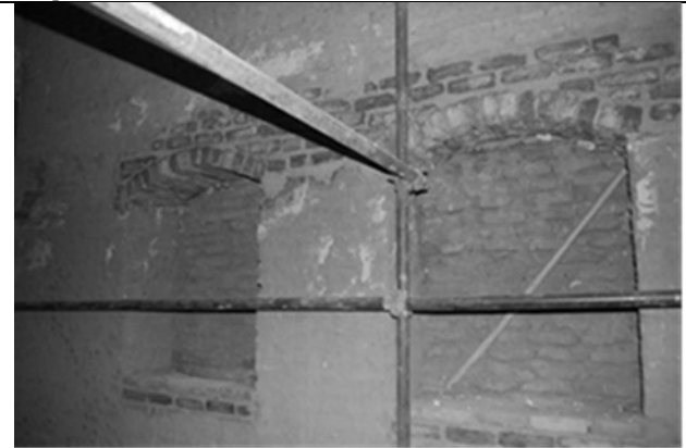
Wall niches changed from a square shape to an arch form in spaces 9 and 10 of Parvin Etesami House.
