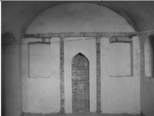
A fireplace that is repaired in underground space number 4 of Parvin Etesami House.
