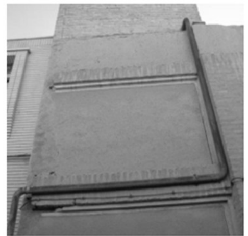
Problem 4: Presence of gas piping and gas valves on the façades. Solution: Creating a gap in the façade and inserting the pipes into it is a definitive solution, and if this is not possible, painting the gas pipes in a colour that matches the façades is a temporary solution.
