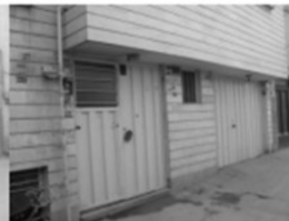
Problem 4: Presence of gas piping and gas valves on the façades. Solution: Creating a gap in the façade and inserting the pipes into it is a definitive solution, and if this is not possible, painting the gas pipes in a colour that matches the façades is a temporary solution.
