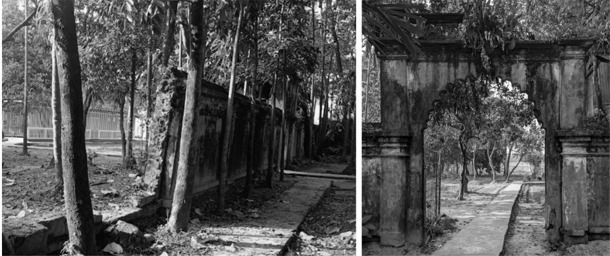
Figure 6. CURRENT CONDITION OF MUGHAL GATE AND ENTRANCE THROUGH IT TO INNER COURT
