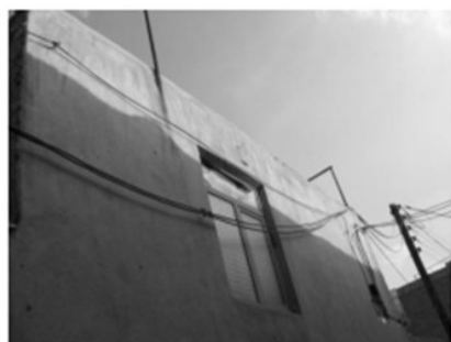
Problem 3: The presence of electric poles and hanging electrical wiring on the façades. Solution: Remove electric poles and design wall lights.
