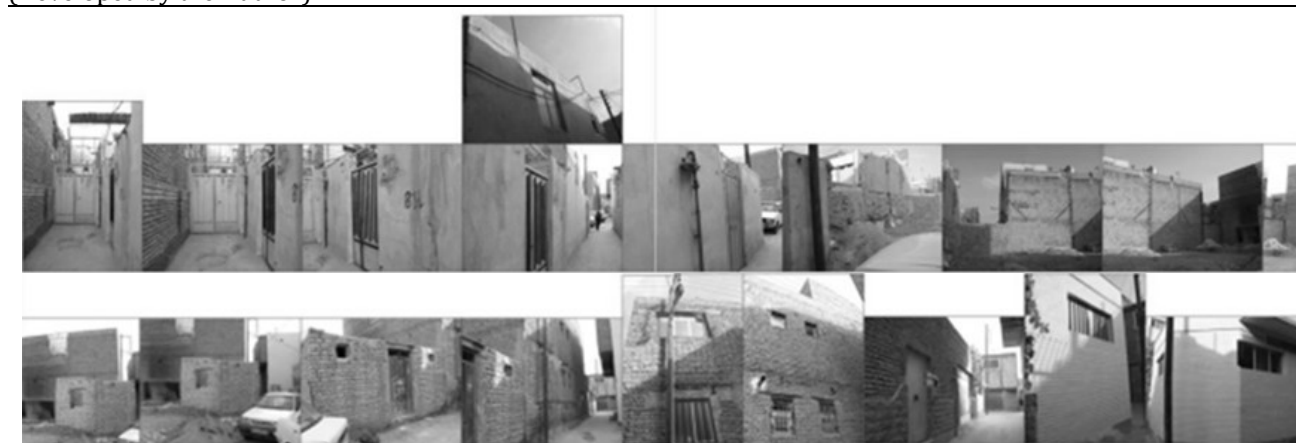
Current Pictures of the Eastern Side of the Passage.
