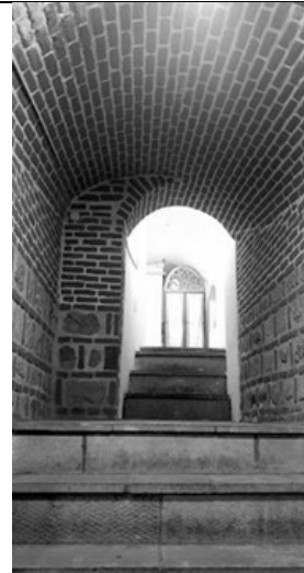
Using stone to reduce the height of the first step in the basement of Parvin Etesami House.
