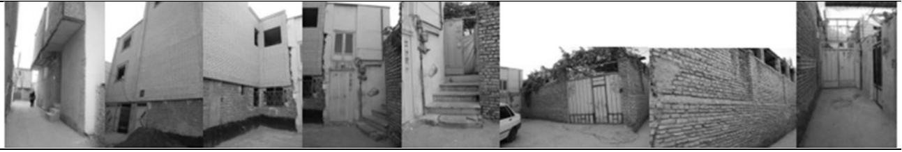
Current Pictures of the Western Side of the Passage.
