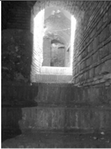
Using stone to reduce the height of the first step in the basement of Parvin Etesami House.
