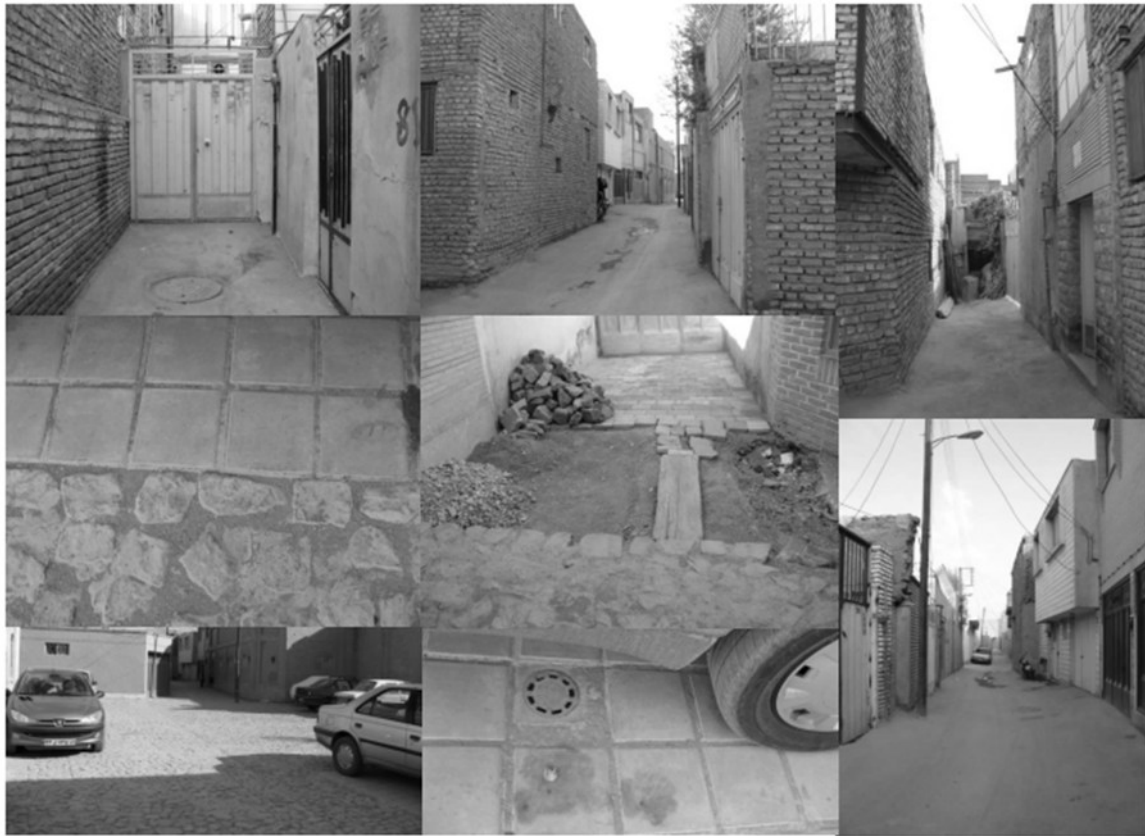
Problem 10: Lack of proper carpet floor design (inappropriate asphalt and carpet floor). Solution: Proper carpet floor design.
