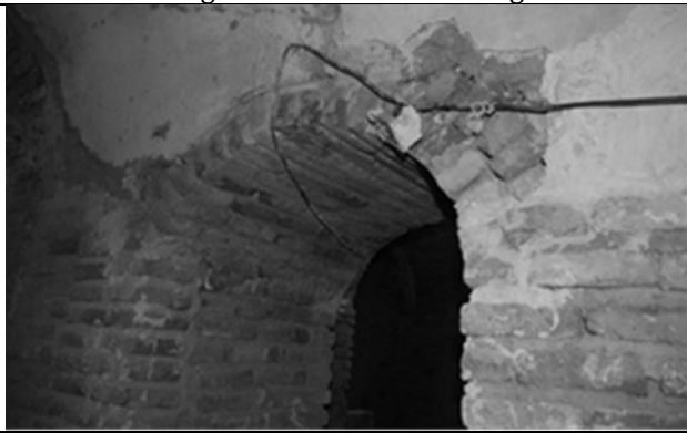
Construction of an arch in the basement of Parvin Etesami House.
