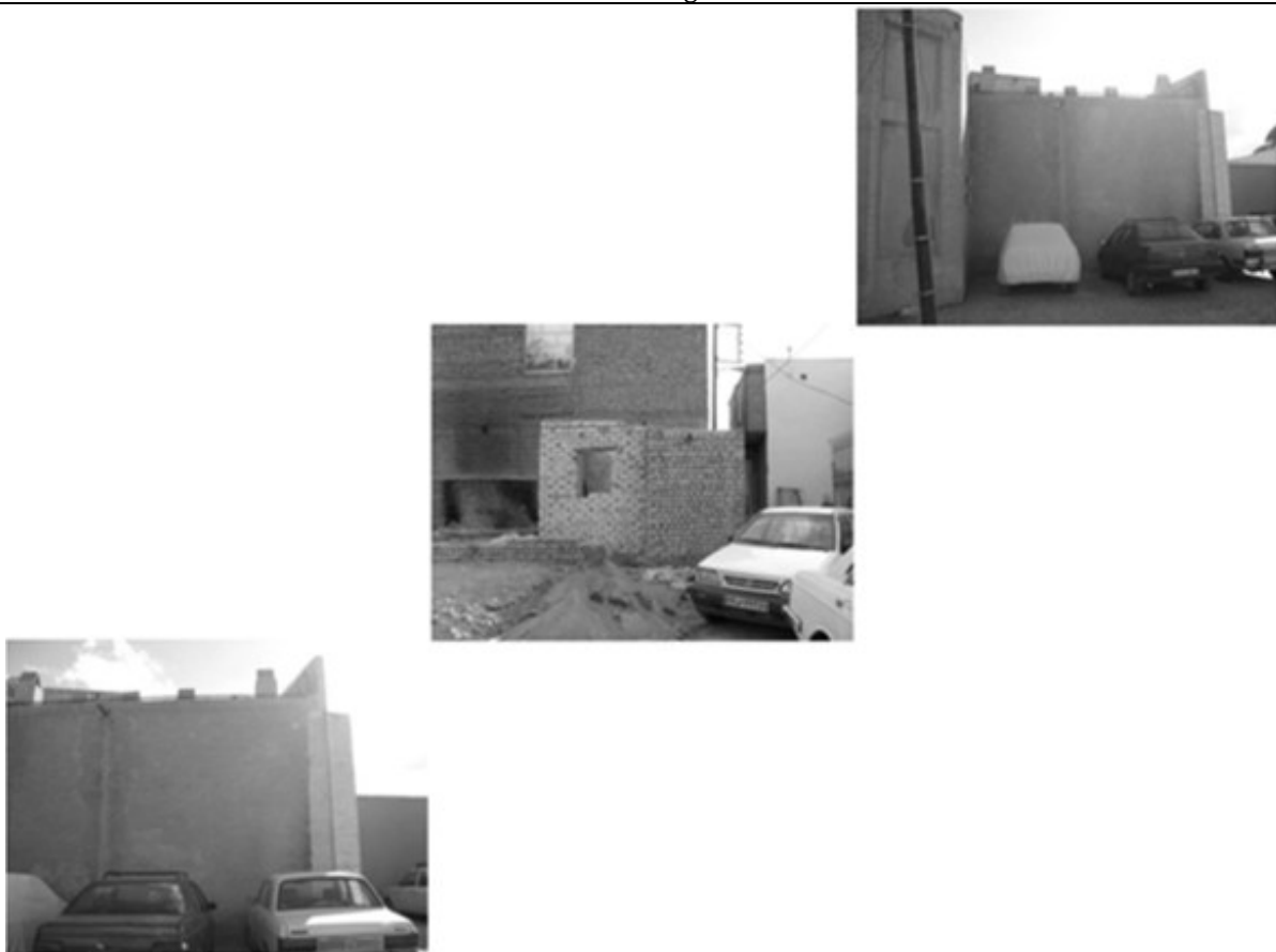
Problem 11: Inconsistency in the brickwork of the façades. Solution: Proper design and implementation of the bricks in the façades.
