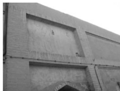
Problem 3: The presence of electric poles and hanging electrical wiring on the façades. Solution: Remove electric poles and design wall lights.
