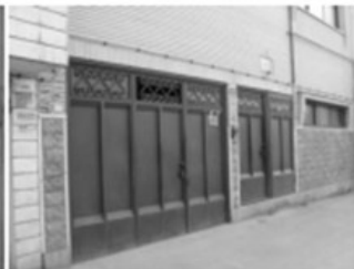
Problem 4: Presence of gas piping and gas valves on the façades. Solution: Creating a gap in the façade and inserting the pipes into it is a definitive solution, and if this is not possible, painting the gas pipes in a colour that matches the façades is a temporary solution.
