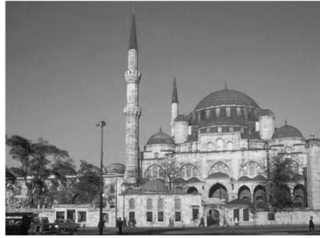
Figure 1. Şehzade Mosque (From: Archnet).
