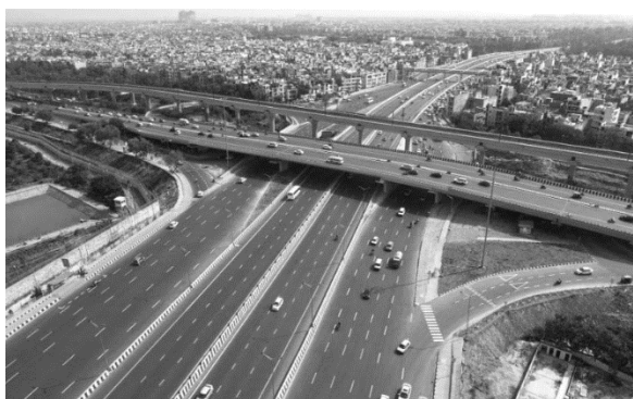
Fig 1. Delhi-Meerut Expressway, the widest expressway in India with 14 lanes
