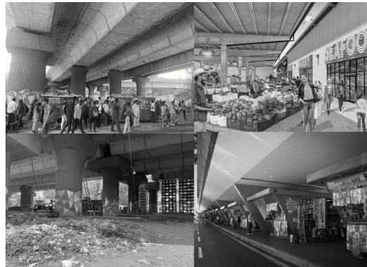
Fig 5. Hebbal Flyover: left-right; existing condition and recommended strategy.
