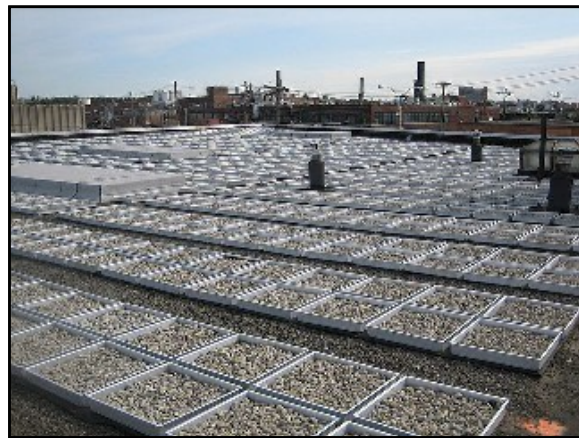
Şekil 8. Mavi Çatı Uygulaması ( https://sustainabletechnologies.ca/home/urban-runoff-green-infrastructure/low-impact-development/blue-roofs/ )
