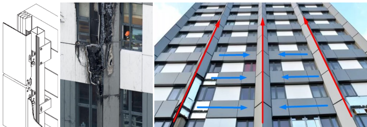
Figure 6. Grenfell Tower façade cladding system with hidden fixings (Symonds, 2021), the burnt cladding and the triangular shaped niches on the facades that pulled the smoke and heat almost like a chimney to the upper floors.
