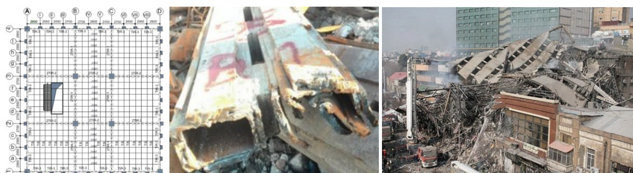
Figure 8. Plasco Tower structural steel plan, the damaged rectangular columns, and the view after the total collapse (Ahmadi, et al. 2019; Macguire, 2017).
