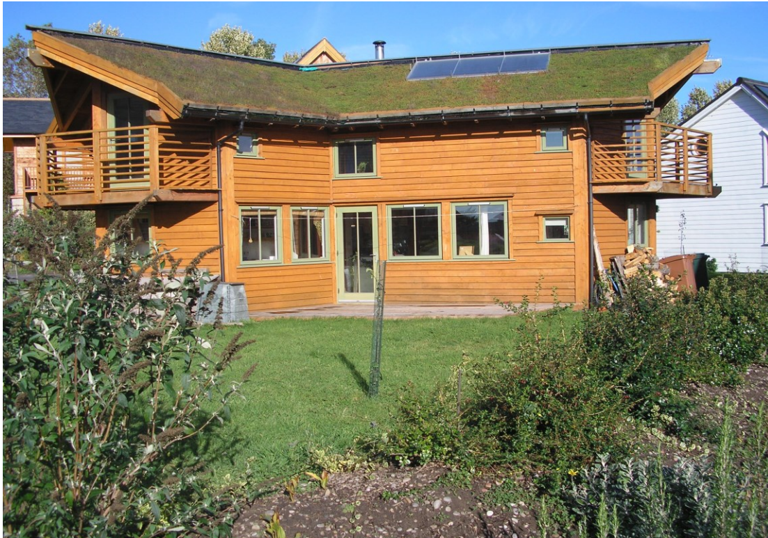
Figure 7. An eco-house at Findhorn Ecovillage with a turf roof and solar panels. https://en.wikipedia.org/wiki/Green_building#/media/File:PA120016.JPG .
